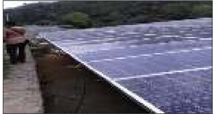
2 MW Canal-top project in Kerala
